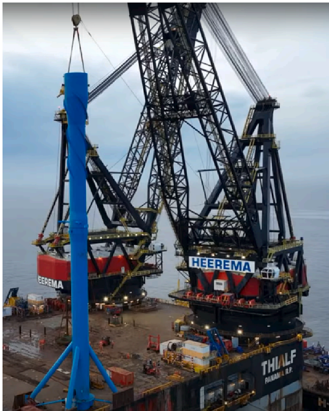
Fig. 3. In-situ installation of the tower with C1 wedge connection [23].
