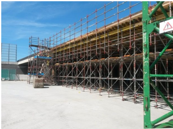
Figure 1 Left: In-Situ concrete deck with false and formwork, right: installation of Prefab box beams
