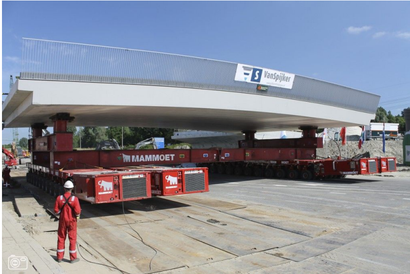
Figure 3-10 Driving a viaduct into place. Courtesy, nufoto.nl
