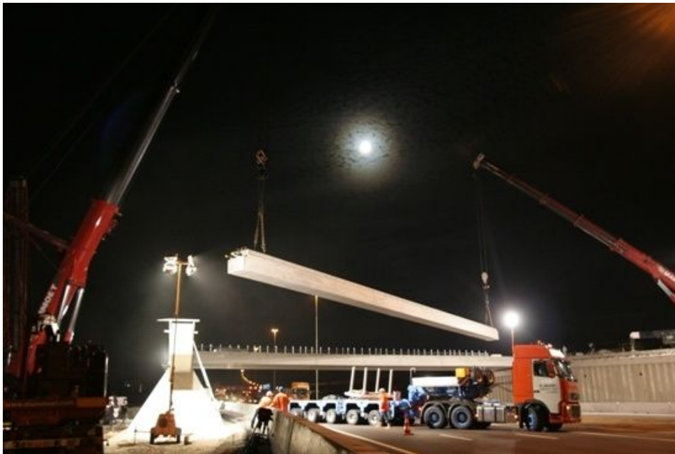
Figure 3-12 Installation of prefab beams, viaduct Lage Weide A2
