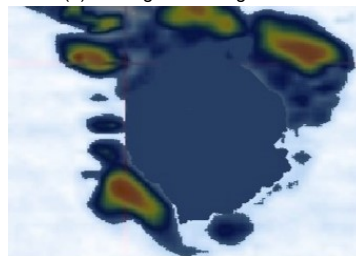
(c) Blend of damaged area
