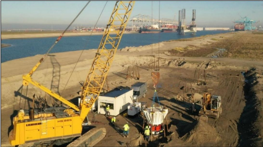
Figure 1: Lifting the load test frame into place at the Amaliahaven test site
