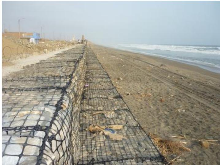
Figure F.2: En example of an application of gabions along the shore. [24]
