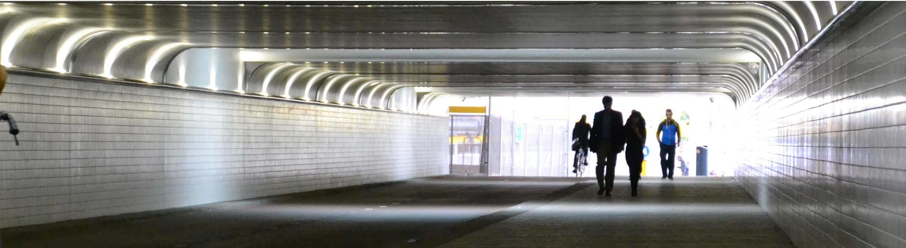
Secondary tunnel in Rotterdam CS
