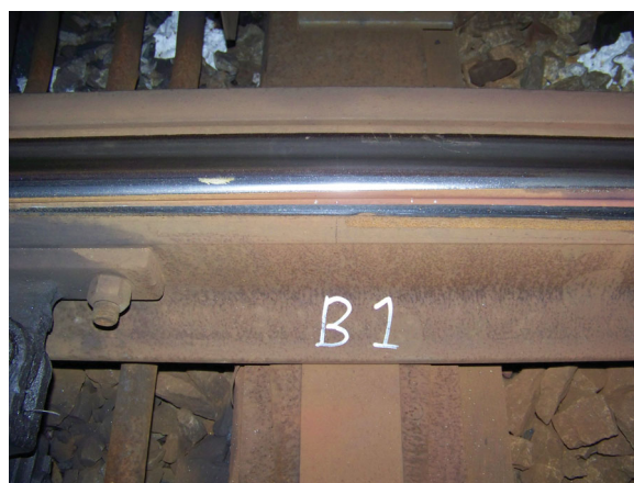
Figure 15. Switch panel of ‘mild’ wearing switch (left switch and stock rail). No wear debris observed. At the gauge face remains of lubrication are present.
