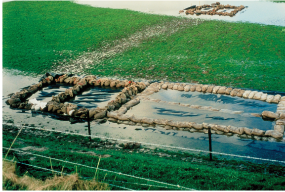
Figure 1.3: Sand boils in 1993 in the Netherlands covered by geotextiles and surrounded by sand bags (source: Beeldbank Rijkswaterstaat)
