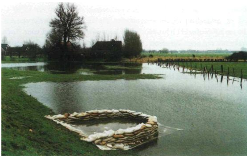
Figure 3.14: Sand bags around a sand boil, source: TAW (1994)
