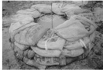
Figure 5.13: Sand bags around an active sand boil (source: Rijkswaterstaat)
