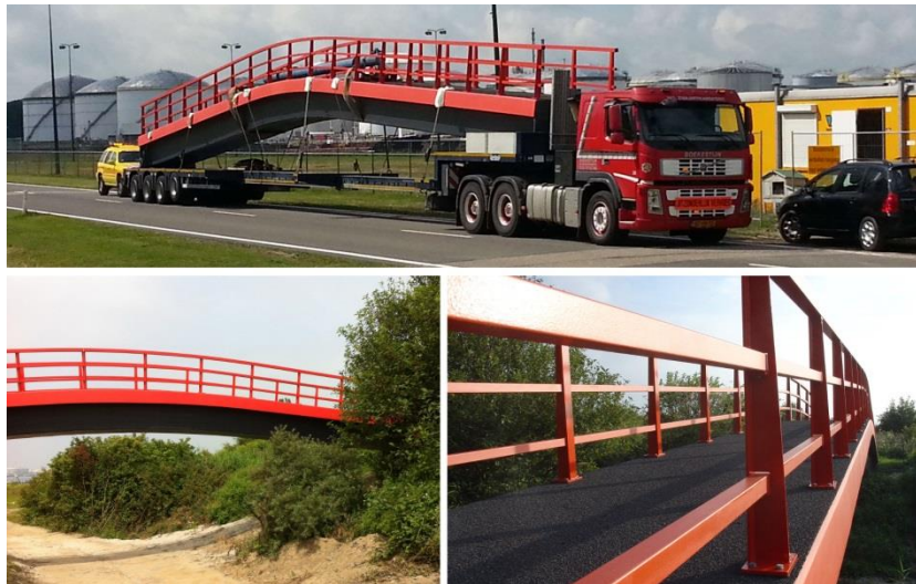
Figure 1.2: a 26 meter long all-GFRP bicycle bridge near Rozenburg, the Netherlands
