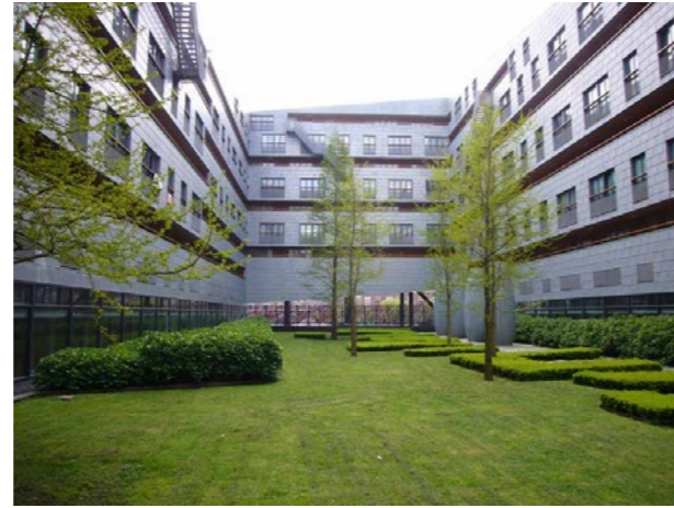
2. The whale housing / de Architekten Cie, Amsterdam, The Netherlands (source: http://openbuildings.com )
