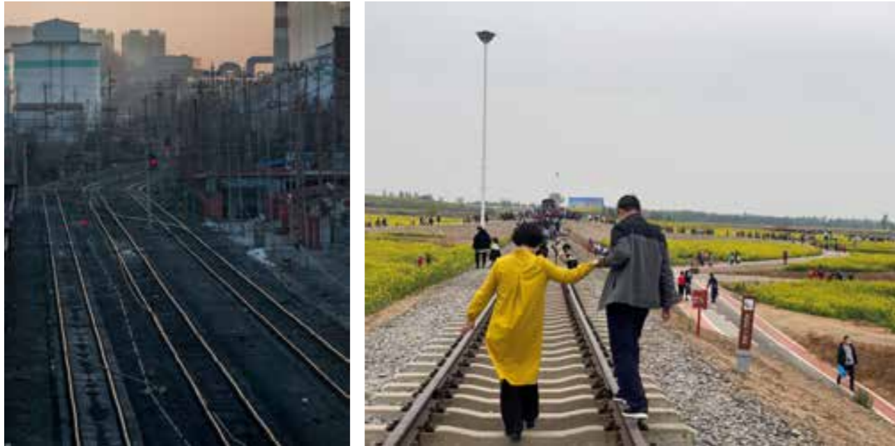
Fig. 6.1.4-6.1.5 Industrial infrastructure Source: author, http://cumbrianrailways.zenfolio.com/img/s/v-3/p205663520-4.jpg
