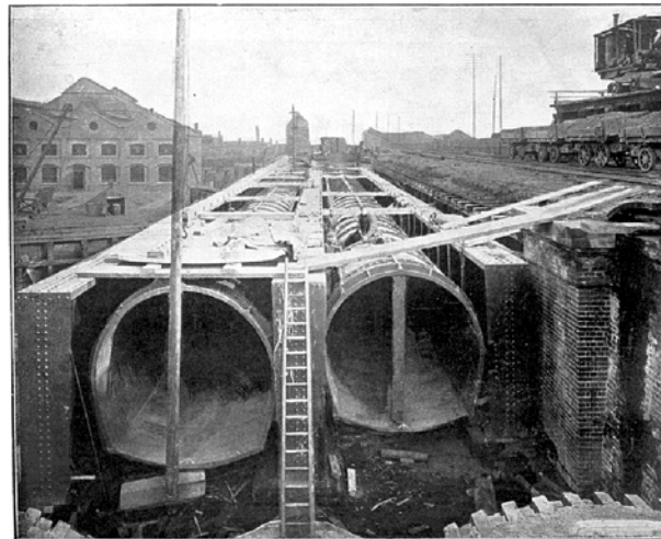
NORTHERN OUTFALL SEWER IN COURSE OF CONSTRUCTION, SHOWING CAST-IRON SEWERS OVER ABBEY CREEK AND CHANNISEA RIVER. 1902-06.
