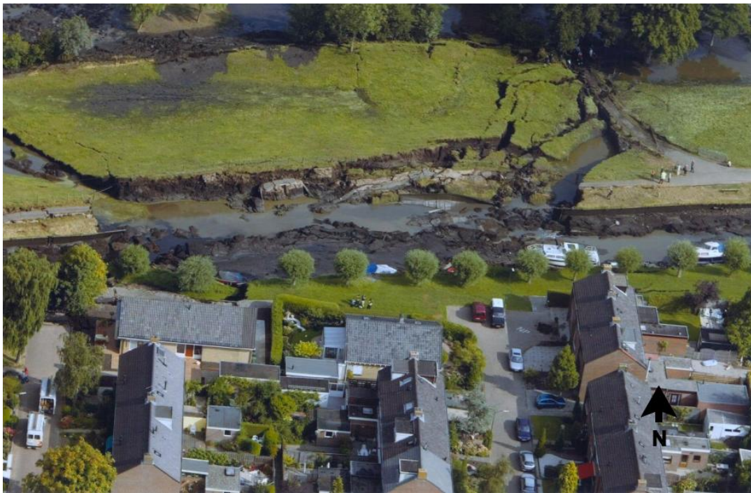
Figure 2.3: Aerial photograph of the breach – north to top (photo from Utrechts Nieuwsblad)
