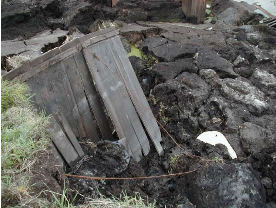
Figure 2.6: Wooden sheet piling of the dike (photo by Ir. J.P. Oostveen )
