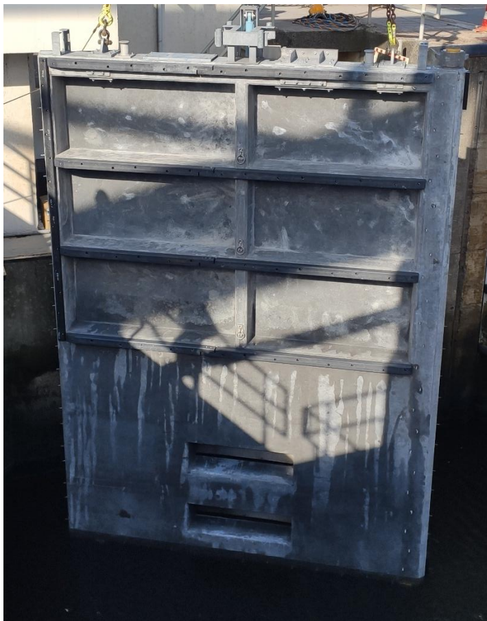
Fig. 8: Photography of the original UHPFRC gate being installed
