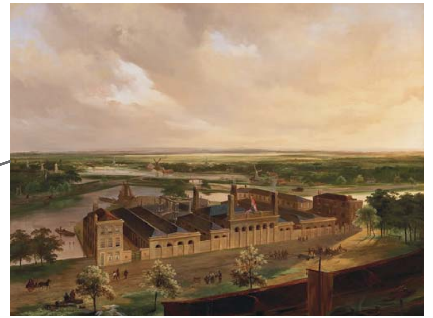
Amsterdamse-Pijp Gas Company, 1826
