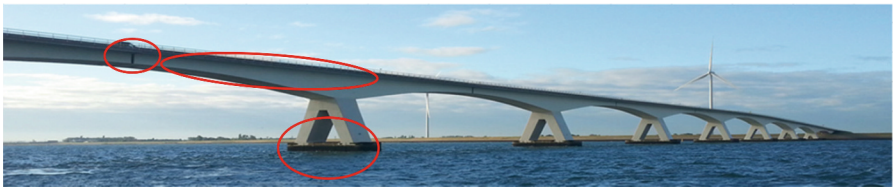
Fig. 1. The Zeeland bridge, showing the locations of main uncertainties.
