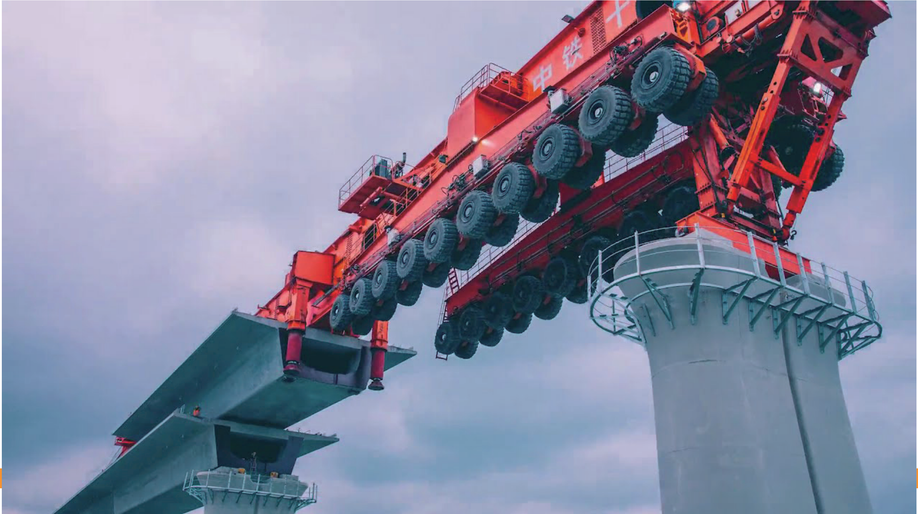
1-16 Girder Kunlun Bridge Erecting Machine (1000t/40m) in use. Photo by Fengle Chen, 2021
