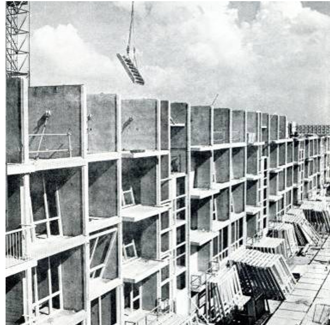
Prefab and assembly of heavy mounting elements
