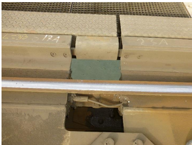
Figuur 13 Lasverbinding in pocket
