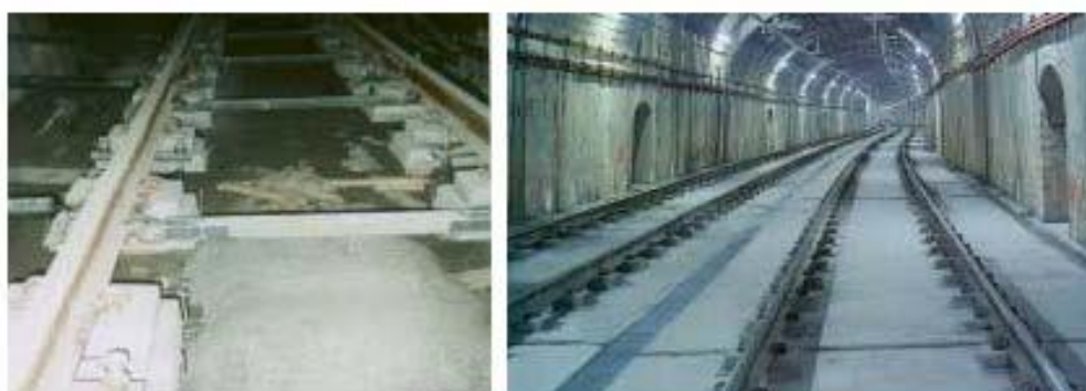
Figure 1 Block track in construction and in use ( Metro de Madrid )
