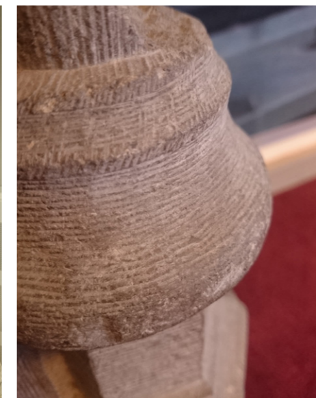
Figure 67. Linear surface indentations on the torus. Source: Author
