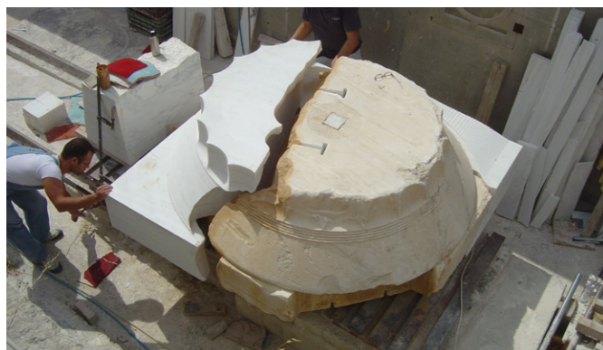
Figure 32. Newly carved Pentelic marble being fitted. Source: YSMA, 2011
