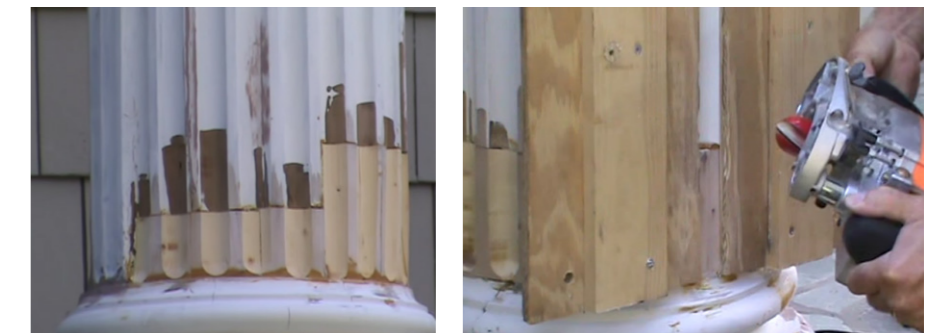
Figure 29. Fluted Wood Column Repair. Source: cunnifjr (Youtube)
