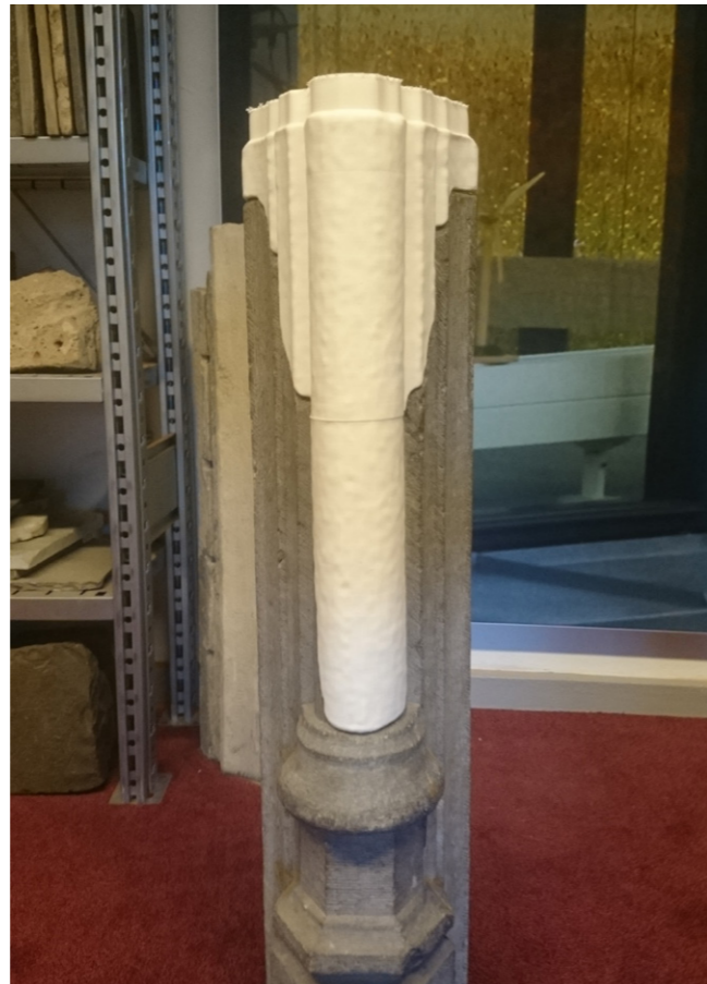
Interestingly, because the manufactured fragment fit the stone column so accurately, it did not require any adhesion or force to be kept in place.
