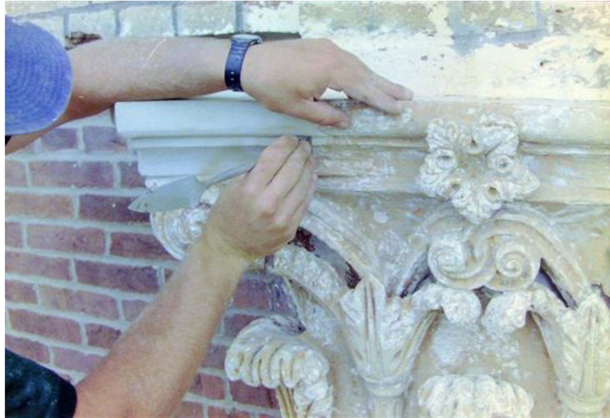
Figure 25. Dutchman Repair of column capital. Source: Schnell Contractors
