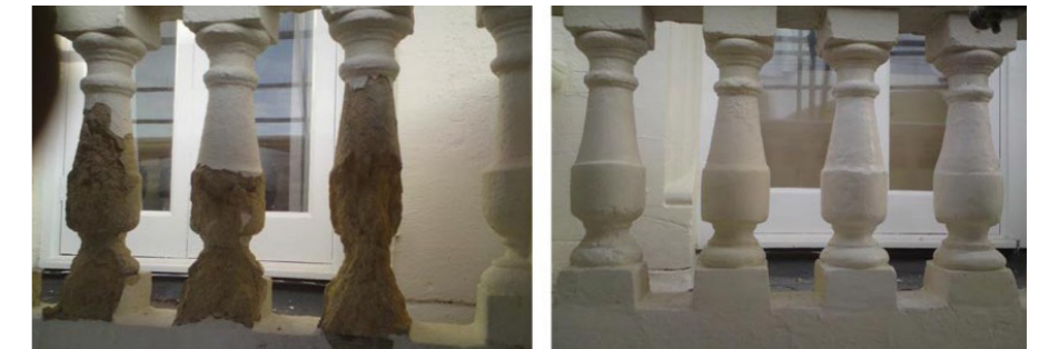
Figure 37. Balustrade Patching (in-situ). Source: Plastic Surgeon Fine Finishers
