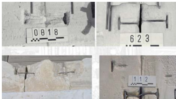
Figure 34. Titanium binding rods. Source: M. Ioannidou, ICOMOS
