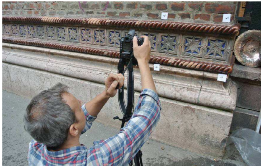
Figure 19. Scanning of tile via Photogrammetry. Source: Adrian Gheorghiu
