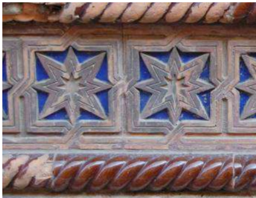
Figure 20. Closeup of Tile. Source: Adrian Gheorghiu
