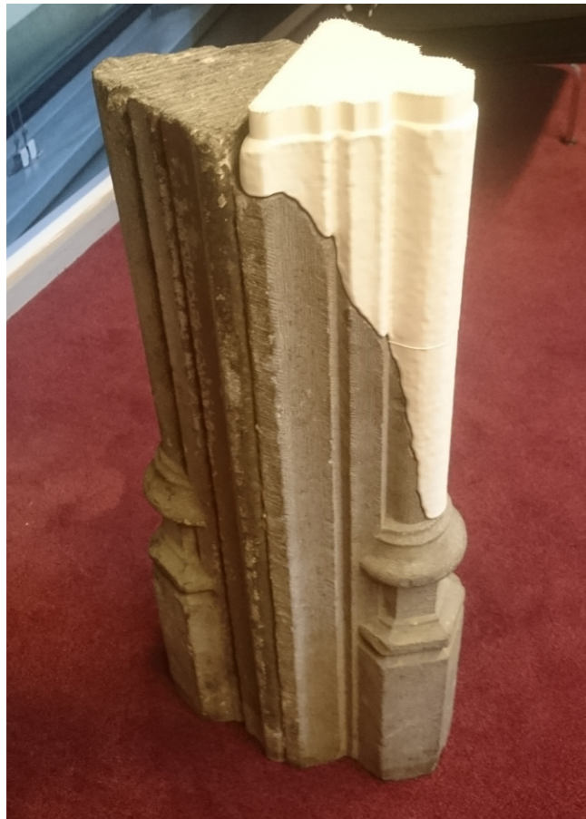
The two printed fragment parts did not need an adhesive to be joined together and would fit together readily.
