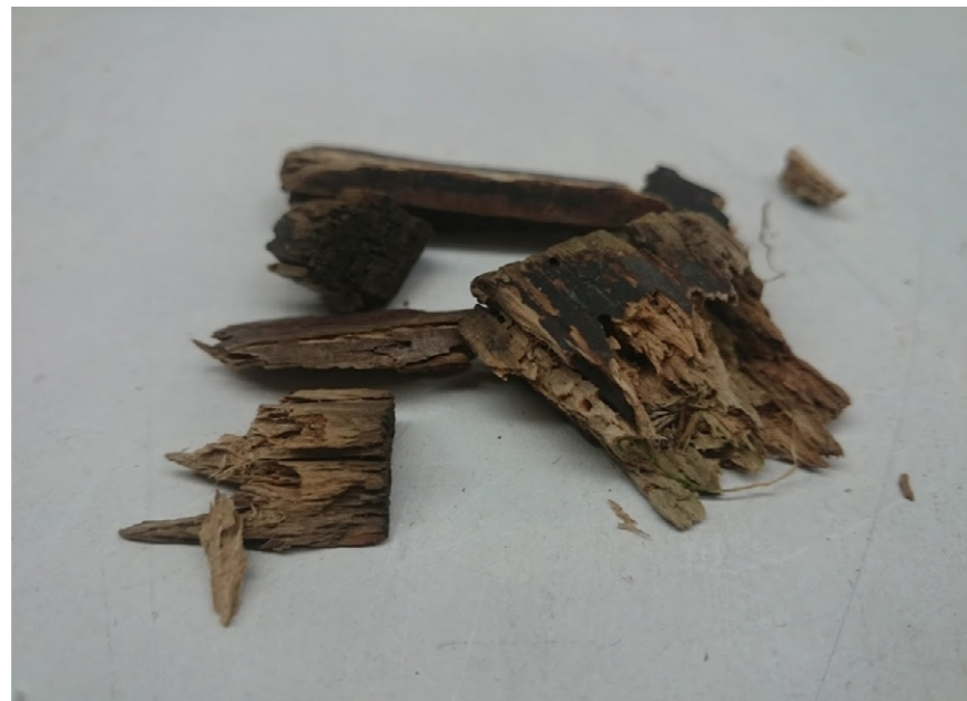
Figure 191. Wood samples with evidence of rot
