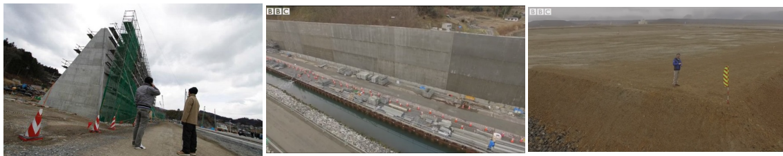
Figure 2.9: Construction of MLS system in Tohoku: Embankments along the coast and ground heightening in the disaster risk zones [BBC, 2016]
