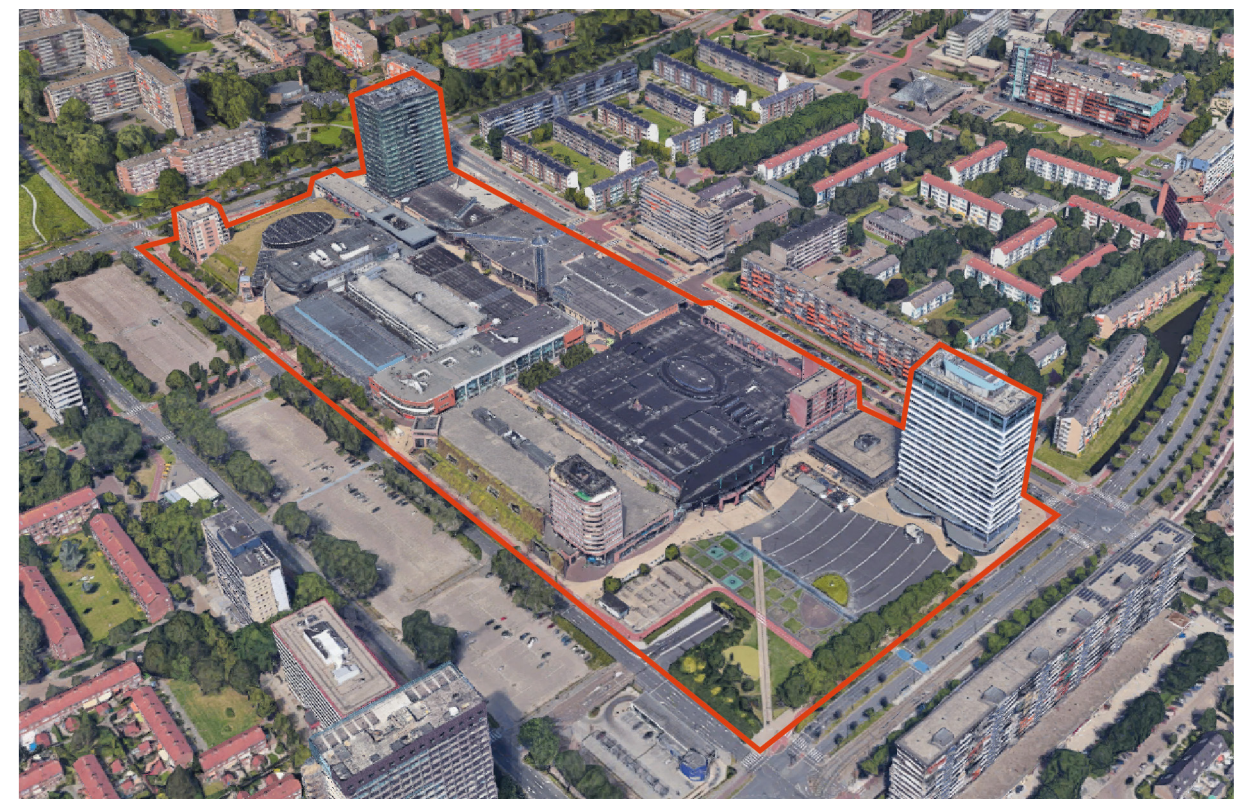
overview of the mall (google)
