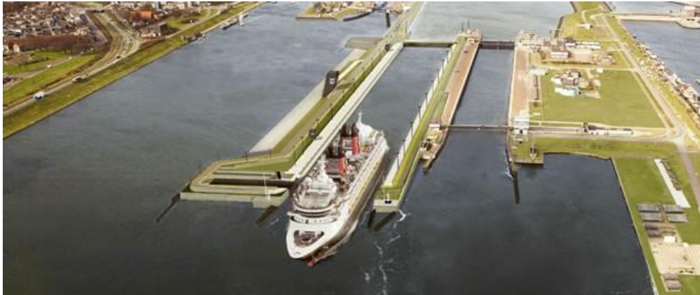
Figure 4.5. New sea lock IJmuiden (RWS, n.a.-b).
