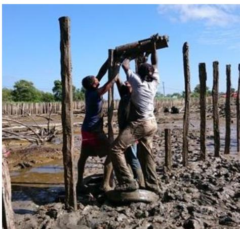
Figure 6.11 Slamming the walaba poles into the soil (Source: Naipal, 2015)
