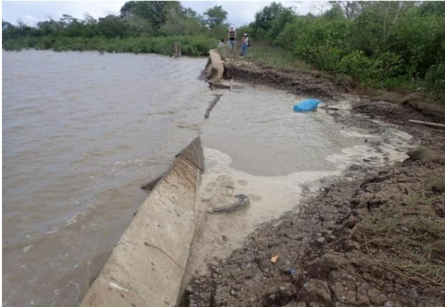
*Figure 2.13 Broken concrete dike (Source: Haage, 2017)*
