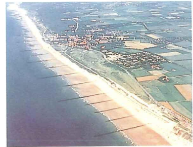
The north-west coast of Walcheren is influenced by sand waves which move along the coast from south to north. This as yet poorly understood phenomenon can lead to fluctuations of tens to hundreds of metres over a period of decades. The dip in a sand wave leads to coastal recession.
