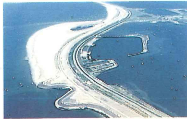
The Brouwersdam. Its construction has stimulated the formation of banks on the outer delta, the "Voordelta".
