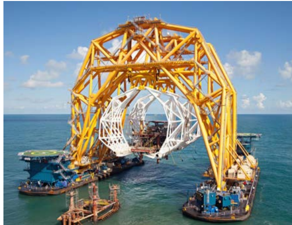
Figure 2.15: Modular topside removal using the Claw [8]
