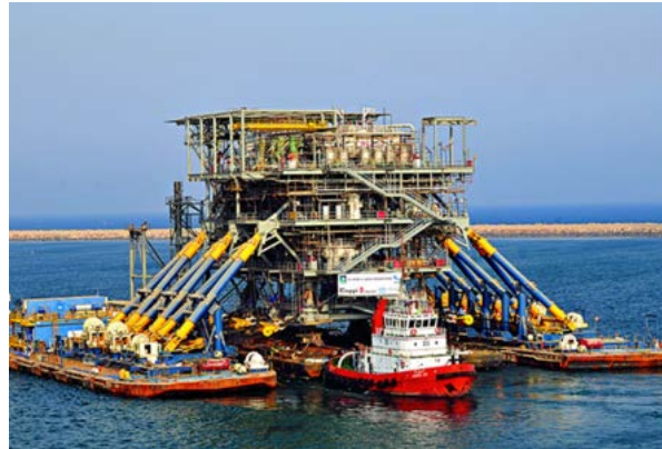
Figure 2.13: The Versatruss lift system installing a topside [? ]
