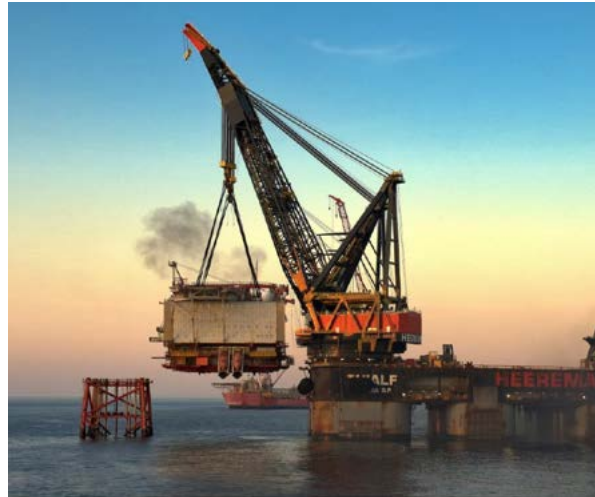
Figure 1.4: SSFV Thialf removing the Jotun B integrated deck in a single piece [26]
