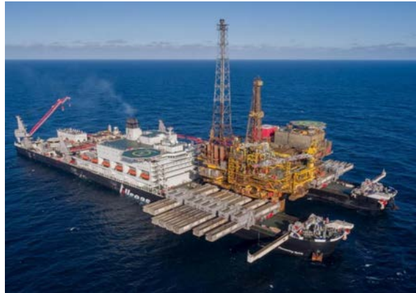
Figure 2.12: Pioneering Spirit after lifting the Brent Delta topside [5]
