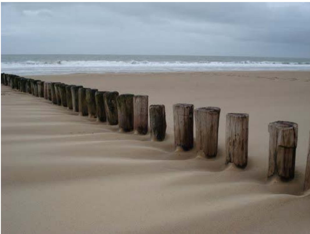
Figure 1.1: Permeable pile groin at Domburg coast (Photo by jwarmelink, www.panoramio.com )
