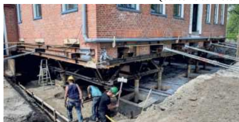
(c) URM monumental building strengthened by means of a 'base isolation'. Source: Dagblad van het Noorden.
