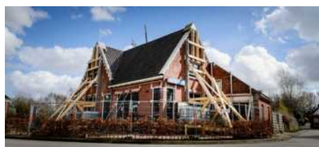
(a) URM residential housing strengthened by means of timber struts. Source: Trouw.
