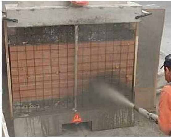
Figure 2.14: Left: application of shotcrete to masonry substrate. Right: details retrofitting approach Shotcrete-URM, [13].
