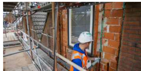
(b) URM residential housing strengthened by means of the QuakeShield. Photo: Archief Huisman Media.
