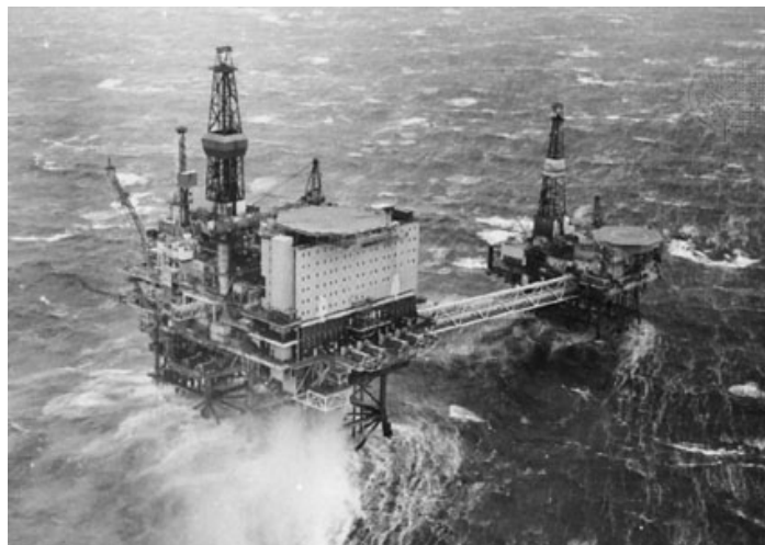
Figure 1-1 Offshore platform under storm conditions in Western Norway
