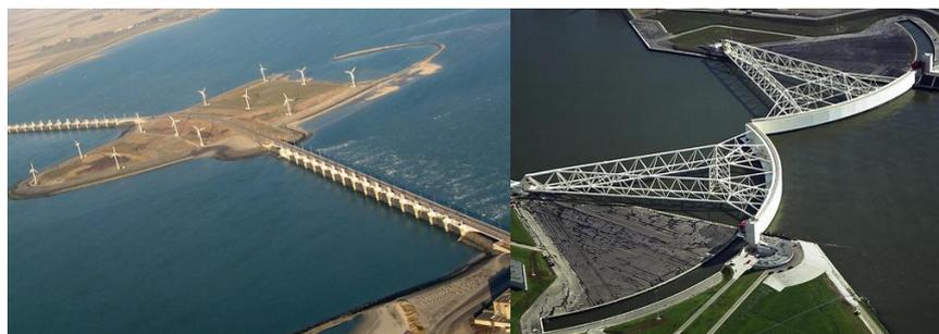
Figure 9- 35. Left: artificial Island in the middle of Eastern Scheldt barrier; Right: chamber of Maeslant barrier built on land
