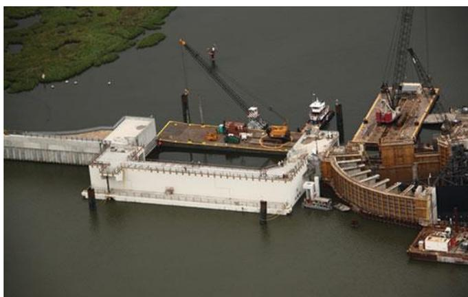
Figure 9- 11. Gulf Intracoastal Waterway Floating Barge Gate made of HPLC
