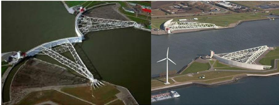
Figure C- 6. Maeslant Storm Surge Barrier, the Netherlands. Left: Closed; Right: Opened.
