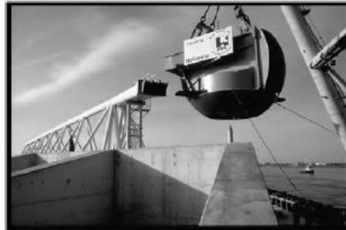
Figure 9- 32. Ball-joint system under construction of the Maeslant barrier(J. P. F. M. Janssen)
