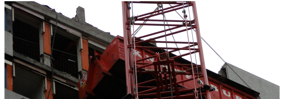
Figure 5 - 10: Demolition process (Knijnenburg, 2010)
