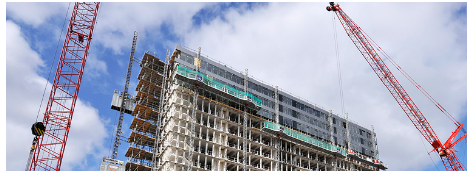
Figure 5 - 7: Assembly on site
