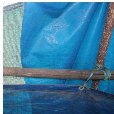
Bamboo connections
