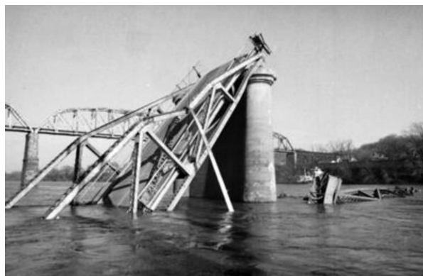
Figure 1.3: The Silver Bridge, which collapsed due to stress corrosion and engineering shortcomings [13].
