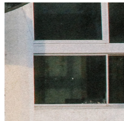
aluminium frame, glass windows additions on the facade
