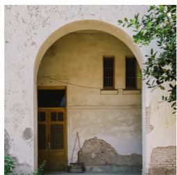
bricks, plaster, and paint for the arches on facade
