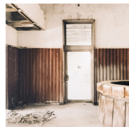
wooden covering on the interior walls
