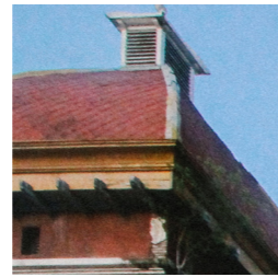
shingle as roofing material of the towers
