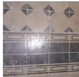
tegel? tiles for the interior area
