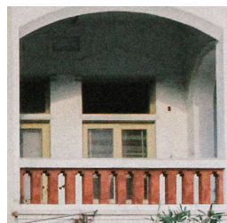
bricks, plaster, and paint for railing on the facade
