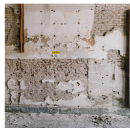
bricks, plaster, and paint on the interior walls
