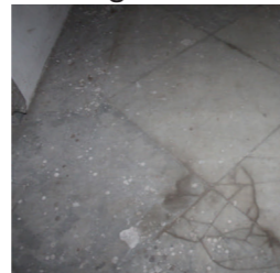
marble floorings on the lobby area
