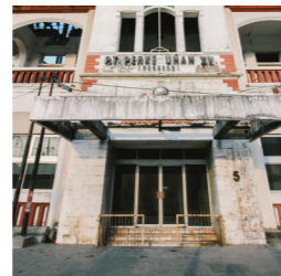
concrete as drop-off roof (additional)
