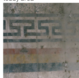
tegel? tiles for the interior area
