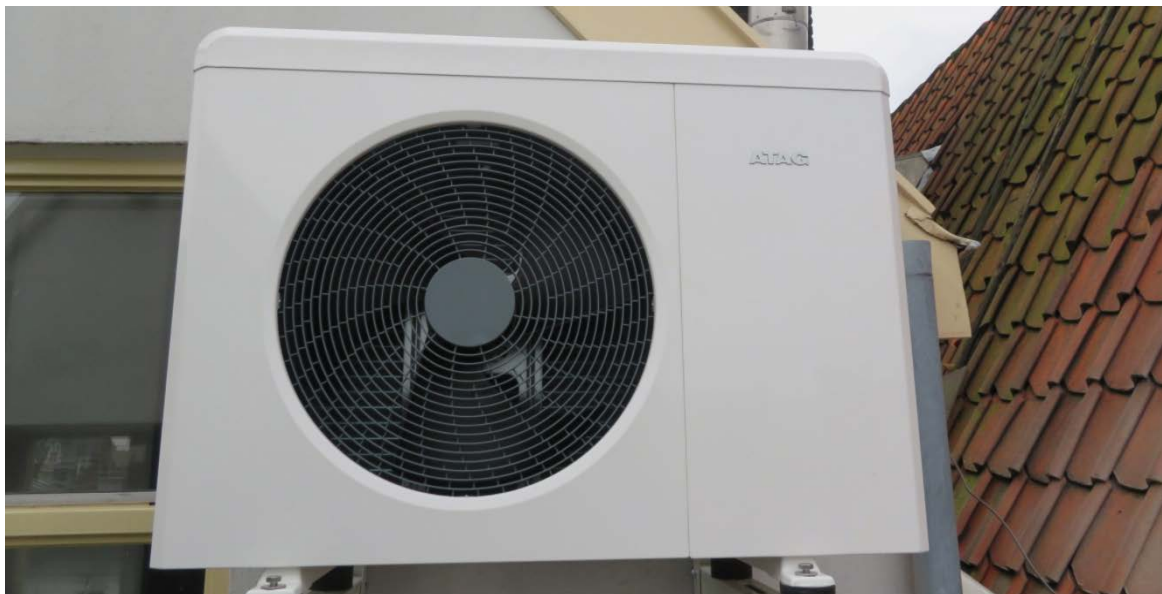
Figure 14: The outdoor unit of the heat pump on the terrace [Foto: De Groene Grachten Amsterdam]
