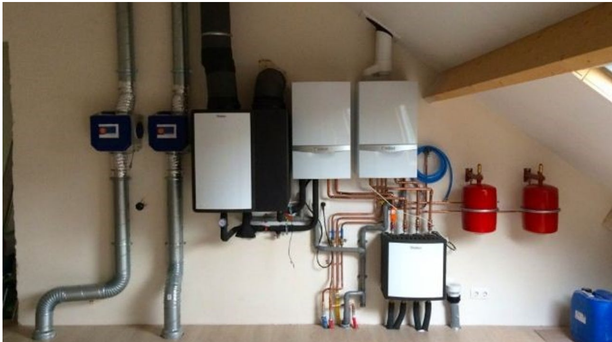
Figure 3: Installation of a hybrid heat pump system; gas boiler, heat pump and hot water storage. [Source: https://www.vakbladwarmtepompen.nl ]
