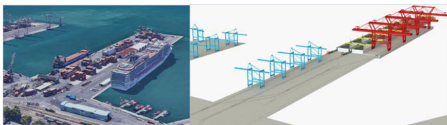
Fig. 9 La Spezia floating port extension
