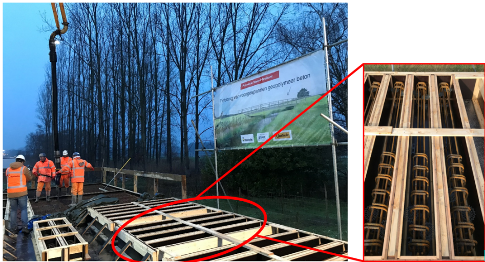
Figure 3.2: Casting of GPC beams at Valkenswaard (Boskalis)
