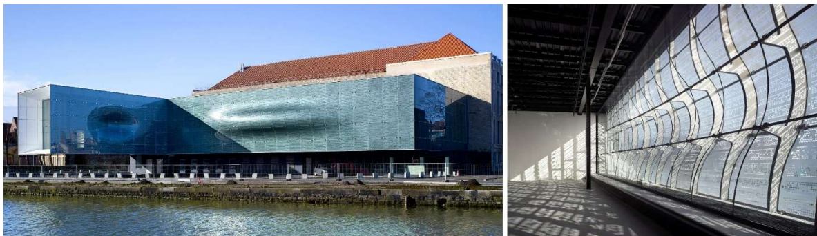
Figure 11 The Fashion and Lace Museum in Calais. (a) The facade consists of double curved glass panels. (b) The panels are joint into a steel structure that followed the panel's profile curves in one direction. Source: < https://www.moatti-riviere.com/en/projects/cultural-space/cite-internationale-de-dentelle-de-mode-calais >
