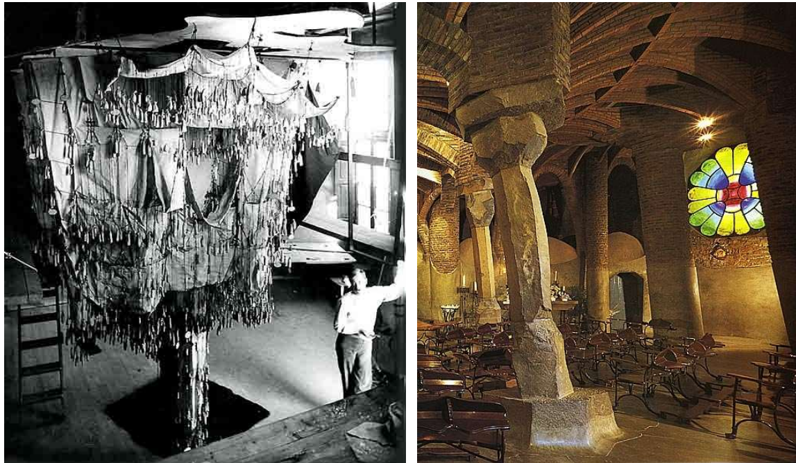
Figure 13 (a) Colonia Guell hanging chain model, (b) the interior Source: < https://structuresandspans.wordpress.com/ >
