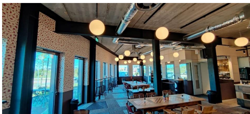
Figure 9: Reused structural steel elements in Biopartner 5 (author)
