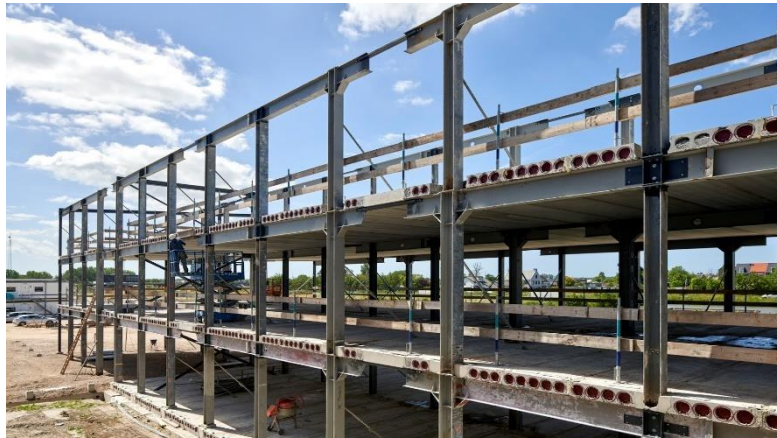
Figure 10: Construction of Biopartner 5 (retrieved from Popma ter Steege Architecten, 2021)
