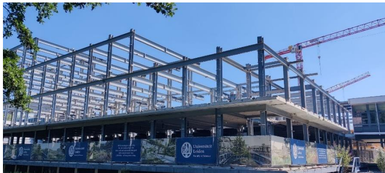
Figure 11: Gorlaeus building – Donor building (author)
