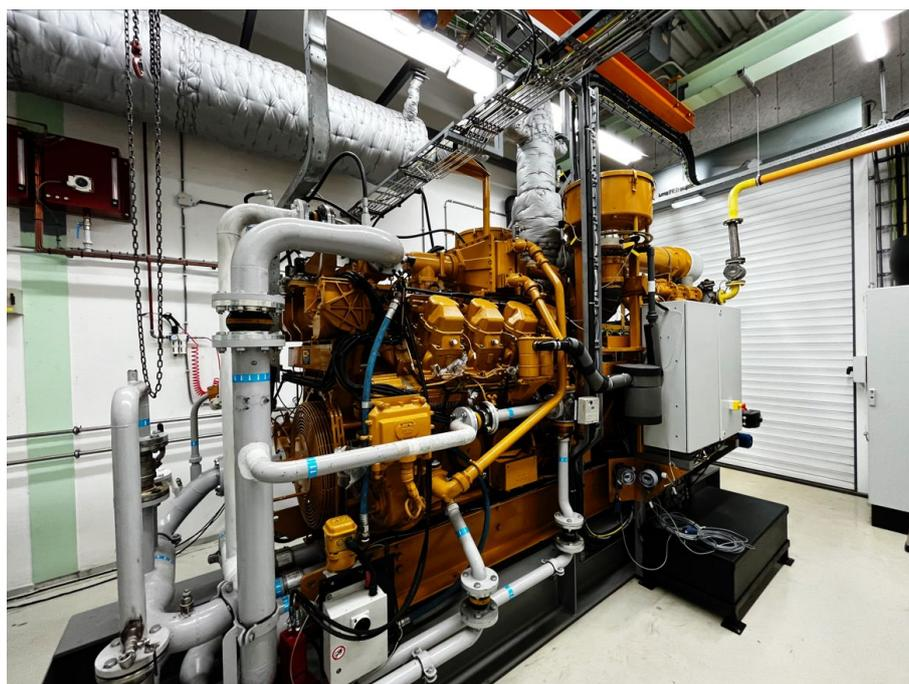
**Figure 1.1:** The CAT G3508A engine installed at the NLDA in Den Helder
