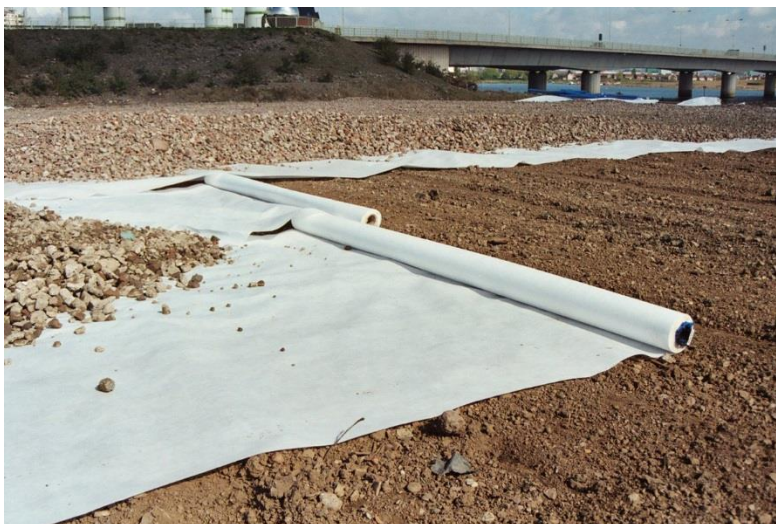
Image 4.4: The white mats are geotextiles used to reinforce soil for construction. Source: dubaicompanieslist.com, 2019.
