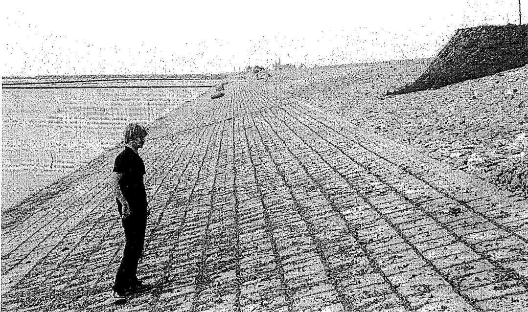
**Figure 4.2** Concrete revetments on a second sea dike in Van Ly.
