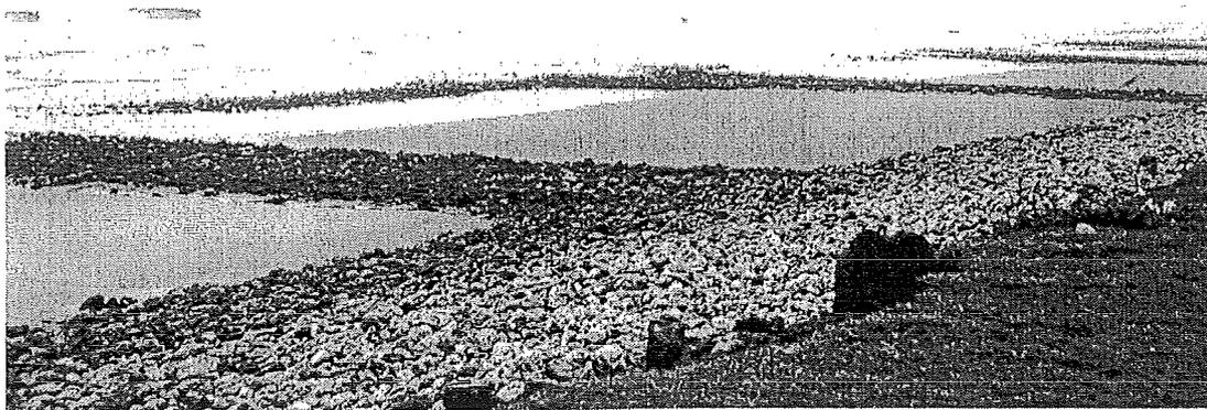
**Figure 4.3** Groins with insignificant impact on the longshore sediment transport at Van Ly beach (photos taken at low water).
