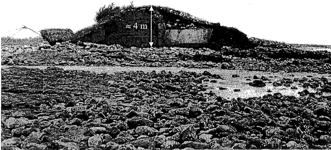
Figure 3.9 Characteristic cross-section of an eroded dike near Van Ly village, (former shrimp farm to the left; open sea to the right).
