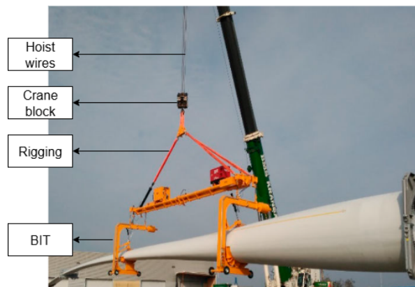
Figure 3.13: Photograph of a turbine blade during lifting. Adapted from Airpes (2025).
