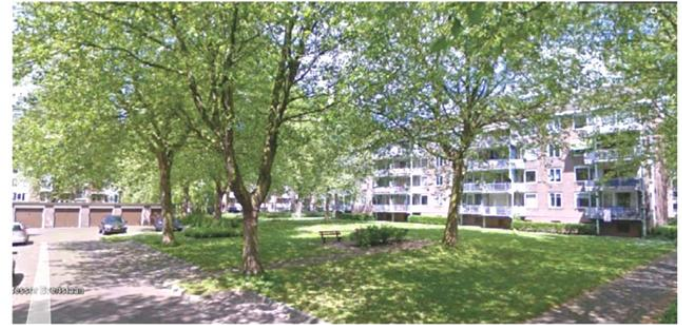
(2) Inner courtyard with grass and benches, garage boxes at the end of the access street
