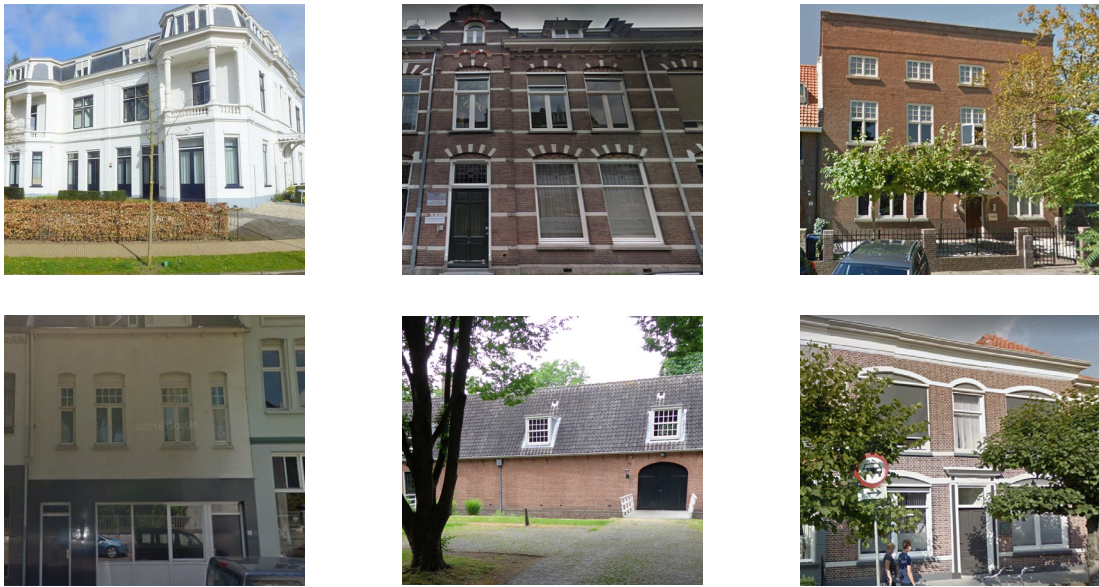
Figure 3.7: ‘Offices’ built before 1950 (Google Street View)
