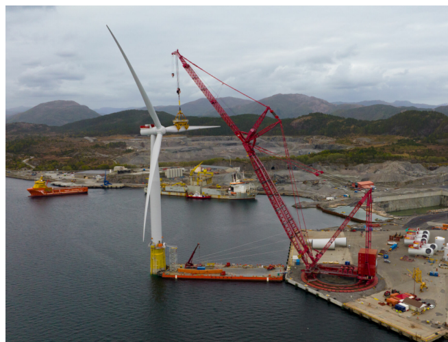
Figure 2.2: Assembly of the Hywind Tampen wind turbines using a spacer barge (Espen Braata, 2022)
