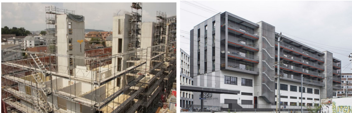
Construction of the concrete stability cores and CLT walls (left) completed building (right). (Source: Burkhalter Sumi)
