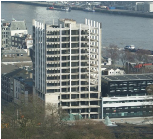
Construction of the extension and reinforcement existing structure (left) and completed building (right)
