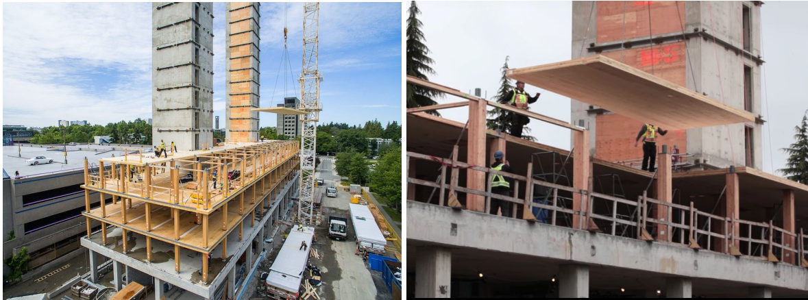
Building in construction (left) and assembly of the floor system through steel connectors (right) (Source: Hermann Kaufmann)
