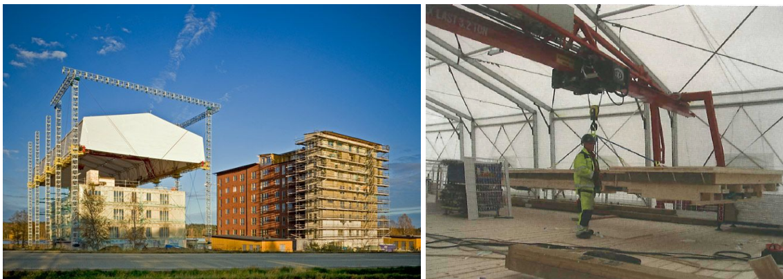
Weather protection system with integrated overhead crane (left) and lifting of prefabricated floor element inside the tent (Source: Johan Vessby)
