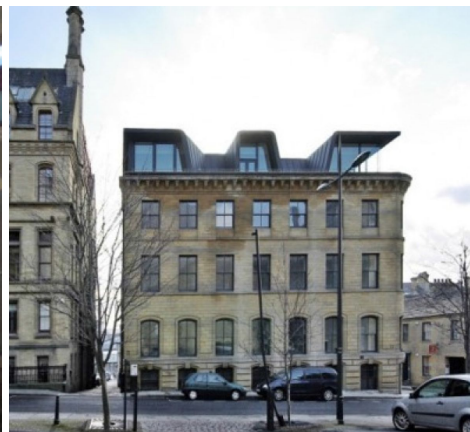
Construction of CLT folded plate (left) and completed extension on top of the existing Victorian building (right) (Source: Kraus & Schönberg)
