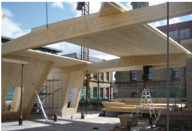
Construction of CLT folded plate (left) and completed extension on top of the existing Victorian building (right) (Source: Kraus & Schönberg)
