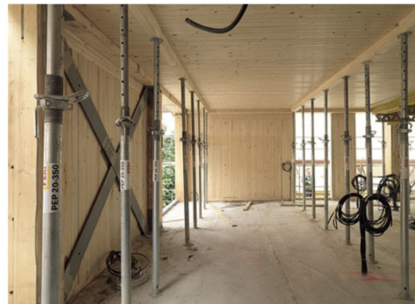
Left, image of post and beams glulam elements with steel connectors. Right, Timber infill panels for compression and steel cross-bracing ties for tension. (Source: Bernd Borchardt)
