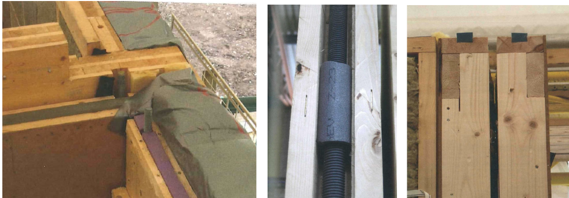
Examples of acoustic detail connections used in Limnologen building. From left to right: Detail at exterior wall; structural tension rod inside wall cavity; and insulation strips on top of pantry wall. (Source: Kirs Järnerö)
