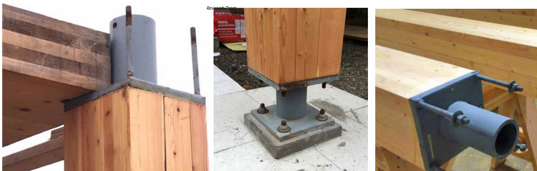
Rounded steel connector detail. (Source: University of British Columbia)
