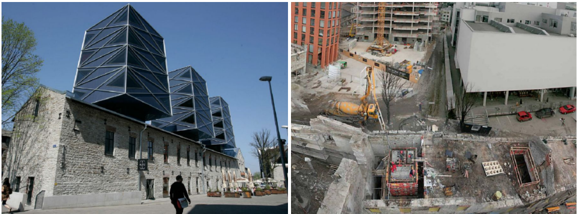
Perspective of completed building (left) and aerial view during construction of concrete cores (right) (Source: KOKO architects)
