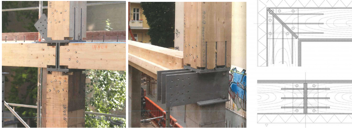
Structural details of steel connector between post and beam timber posts. From left to right, detail normal connection, detail at corner of the building, and technical detail drawings.
