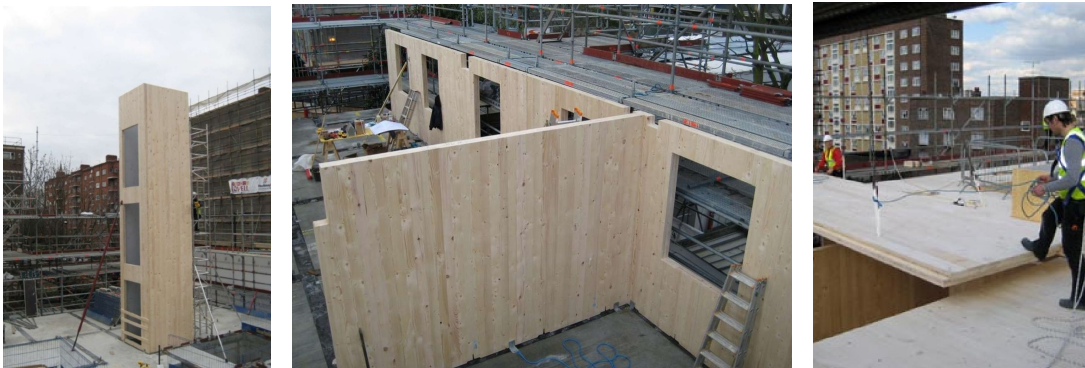
Erection sequence. From left to right, core, shear walls, and floor panel installation (Source: KLH-UK)
