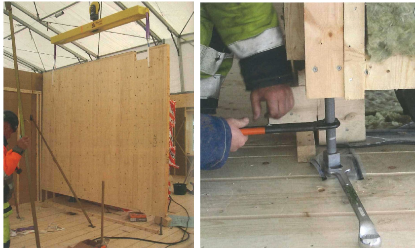
CLT interior wall lifted into place over steel tension rod (left) and interconnection of tension rods between floors (right) (Source: Kirsi Jarnerö)
