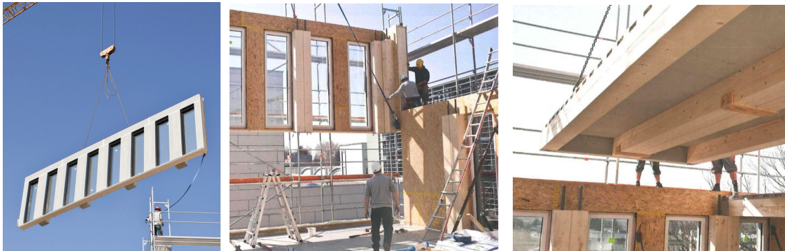
Pictures of the assembly process. From left to right, Lift of façade component, installation façade component, installation floor component. (Source: Architekten Hermann Kaufmann)
