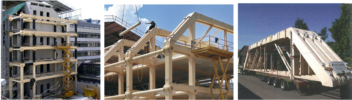
From left to right. Second frame placed into position and braced with oval elements. Bracing of roof trusses. Transport of prefabricated roof truss elements to site. (Source: Blumer Lehmann AG)
