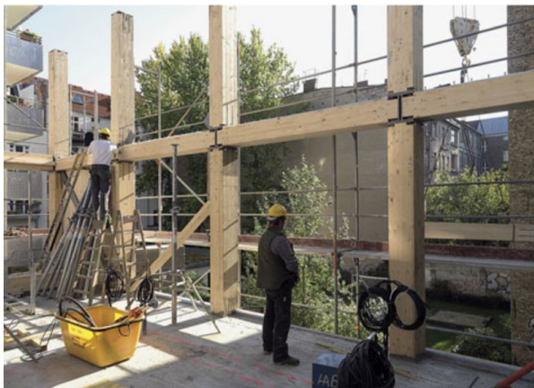
Left, image of post and beams glulam elements with steel connectors. Right, Timber infill panels for compression and steel cross-bracing ties for tension. (Source: Bernd Borchardt)
