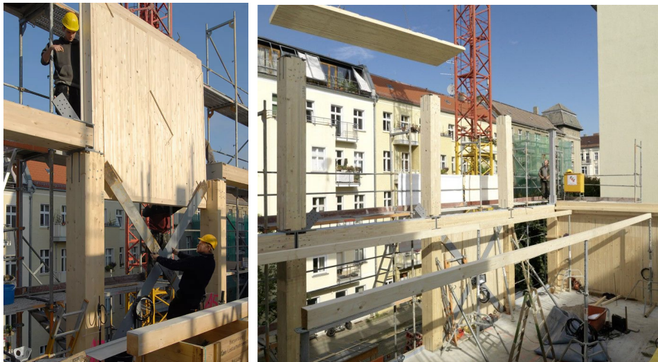
Insertion of infill timber panels (left) and placement of timber floor (right). (Source: Bernd Borchardt)
