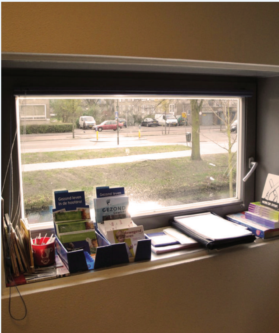
10E. Objects located in windowsill obstruct opening of window.
