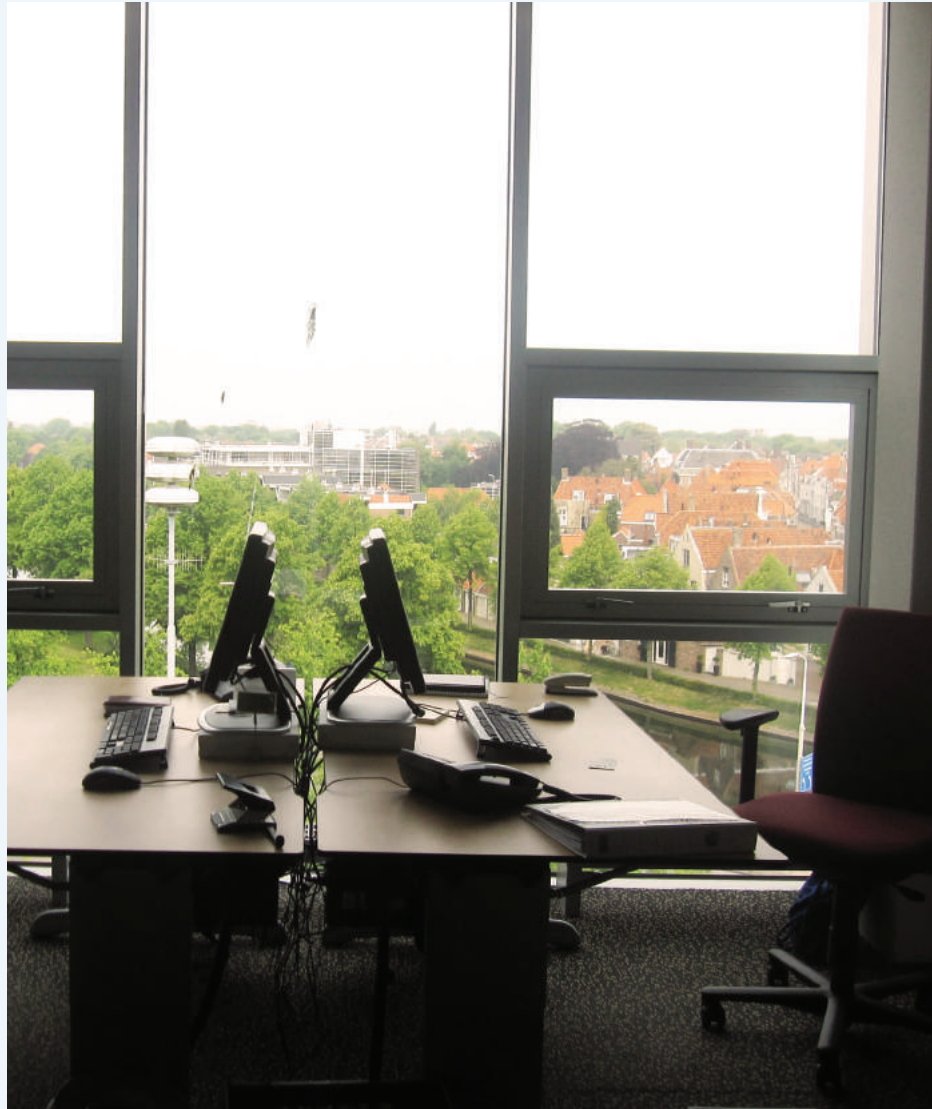
5E. Hardly controllable operable window (top hung outwards opening), only operable in one way at one level.
