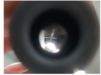
Figure D.4: The the duct inside the manifold. It can be seen that the sensor slightly protrudes from the duct wall.
