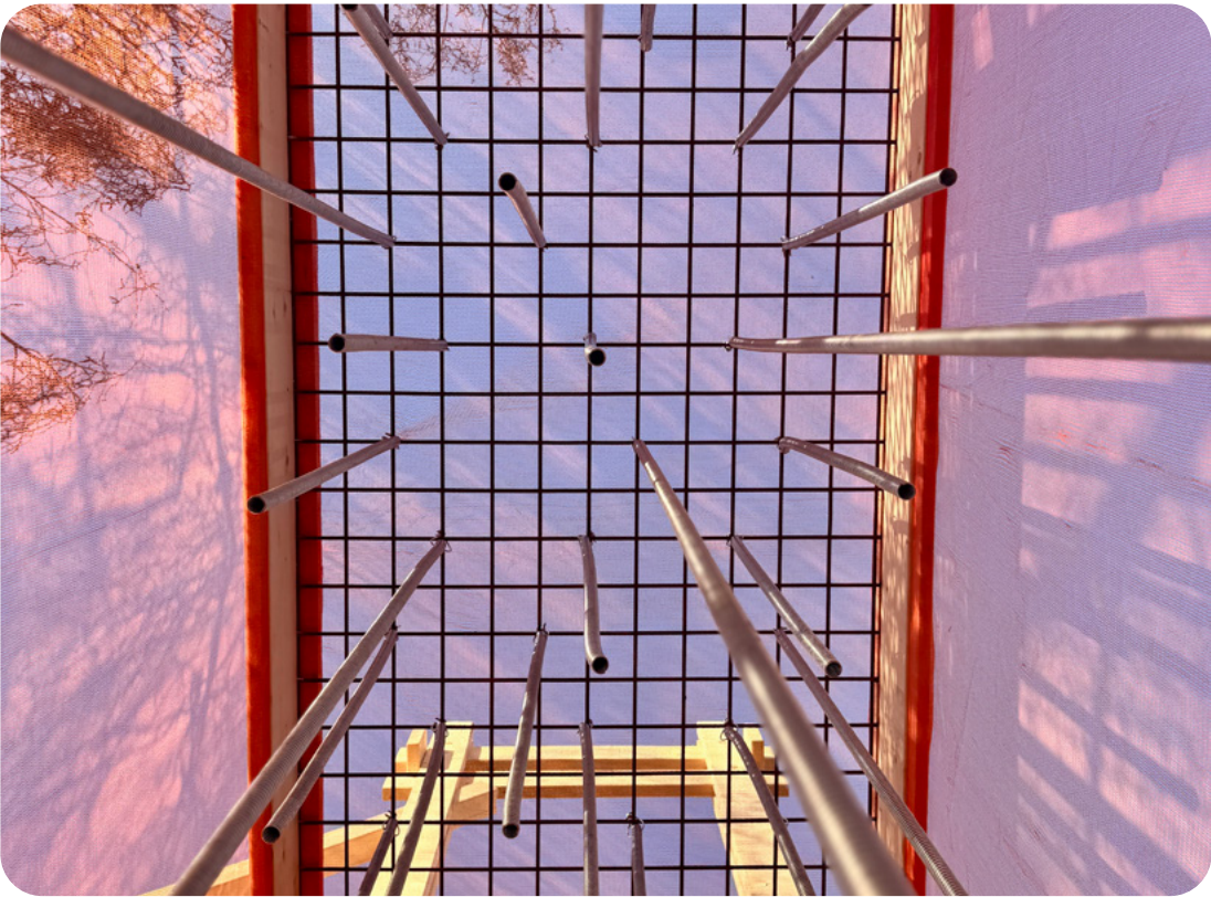
View of Construction at Site 4016. Photographer: Siri Pedersen
